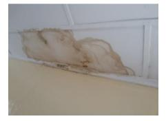
Stained ceiling board due to leaking roof
