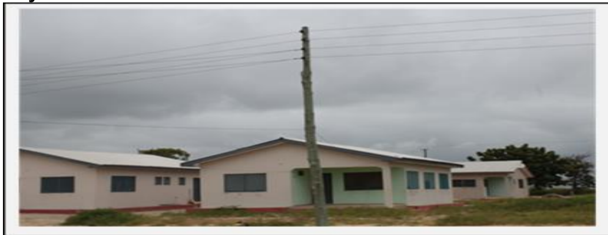
Figure 4: Extension of Electricity Grid to the Keta Sea Defence Resettlement Project
