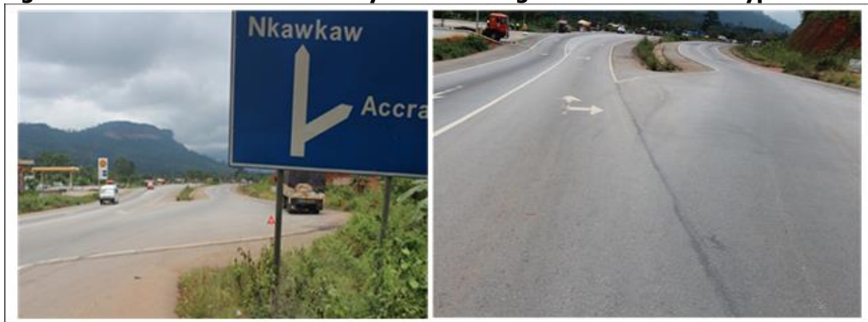
Figure 5: Rehabilitation of the Anyinam-Konongo Road-Nkawkaw bypass
