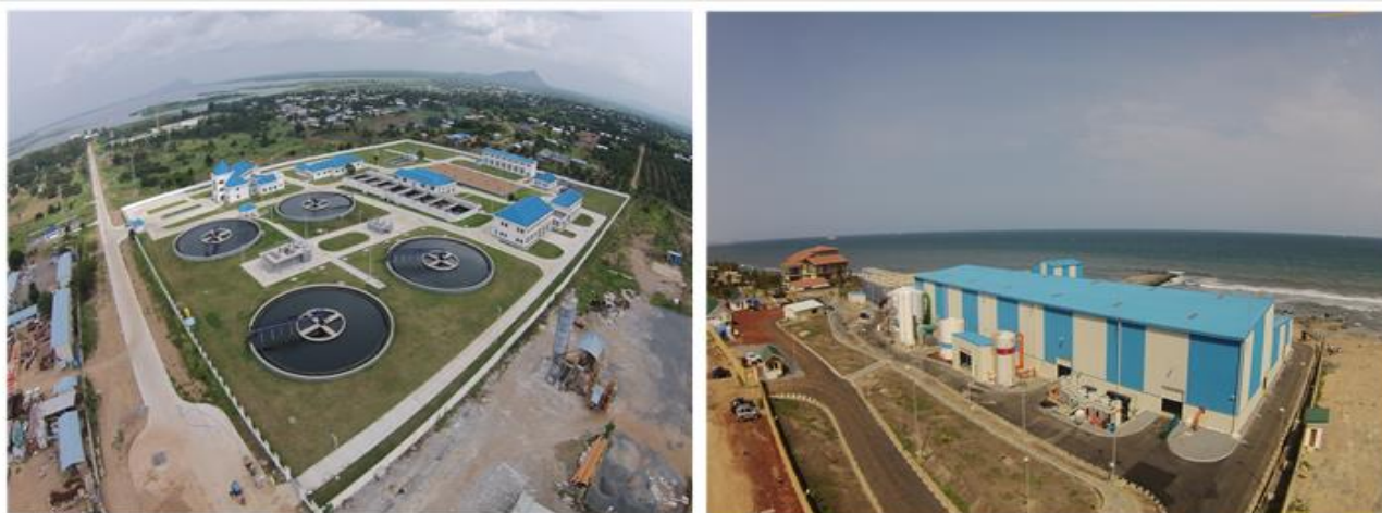
Figure 6: Kpong Water Expansion Project and the Teshie Nungua Water Desalination Plant
