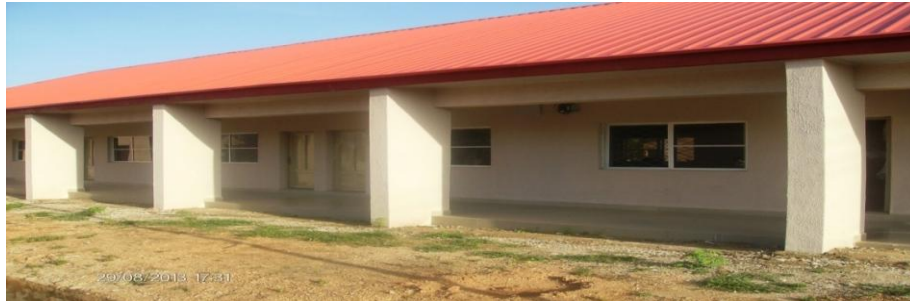
Picture 21: Completed Block of offices for the Faculty of Engineering and Technology
