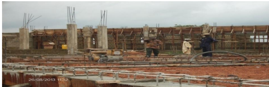
Picture 24: Setting of beams and DPC works for Department of Building Technology in progress at the Polytechnic site.
