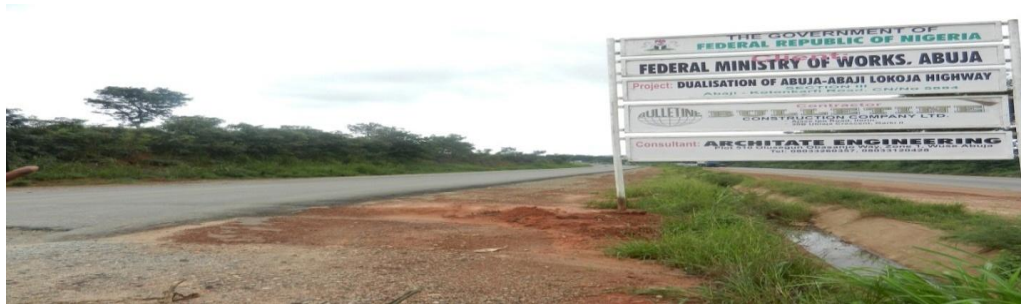
Picture 2: Newly Constructed Portion at Km 0 of the Dualization of Abuja - Lokoja Road Section III (Abaji – Kotonkarfi)
