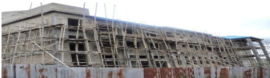
Picture 20: Admin building/Training Centre at roofing level
