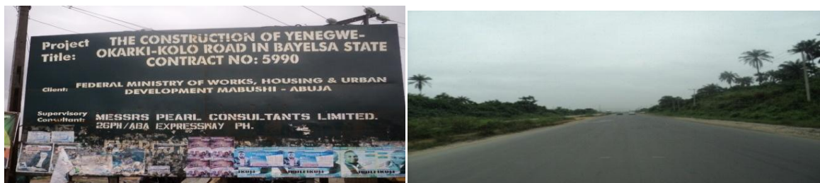
Picture 6: Construction of Yenegwe-Okaki-Okolo road in Bayelsa
