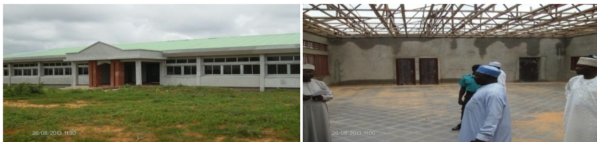
Picture 23: On-going Construction of the Department of Architectural Technology building & the area affected by storm being re-roofed.
