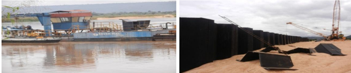
Picture 12: One of the Dredging boats, a completed key wall and vibrator at River Port Lokoja
