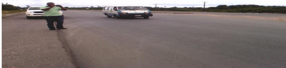
Picture 35: A portion of road completed at Owerri- Elele in Imo State
