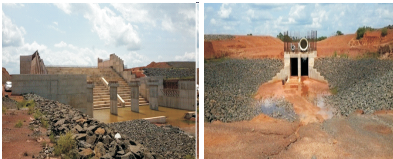
Picture 8: Precast Elements /Spillway Channel at Otukpo Multi-Purpose Dam
