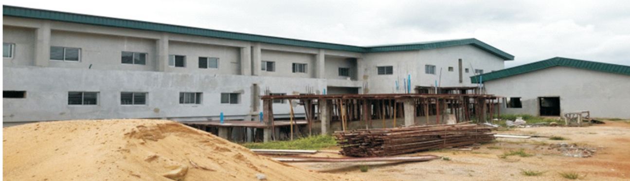
Picture 32: Radiotherapy Complex almost Completed at National Hospital, Abuja
