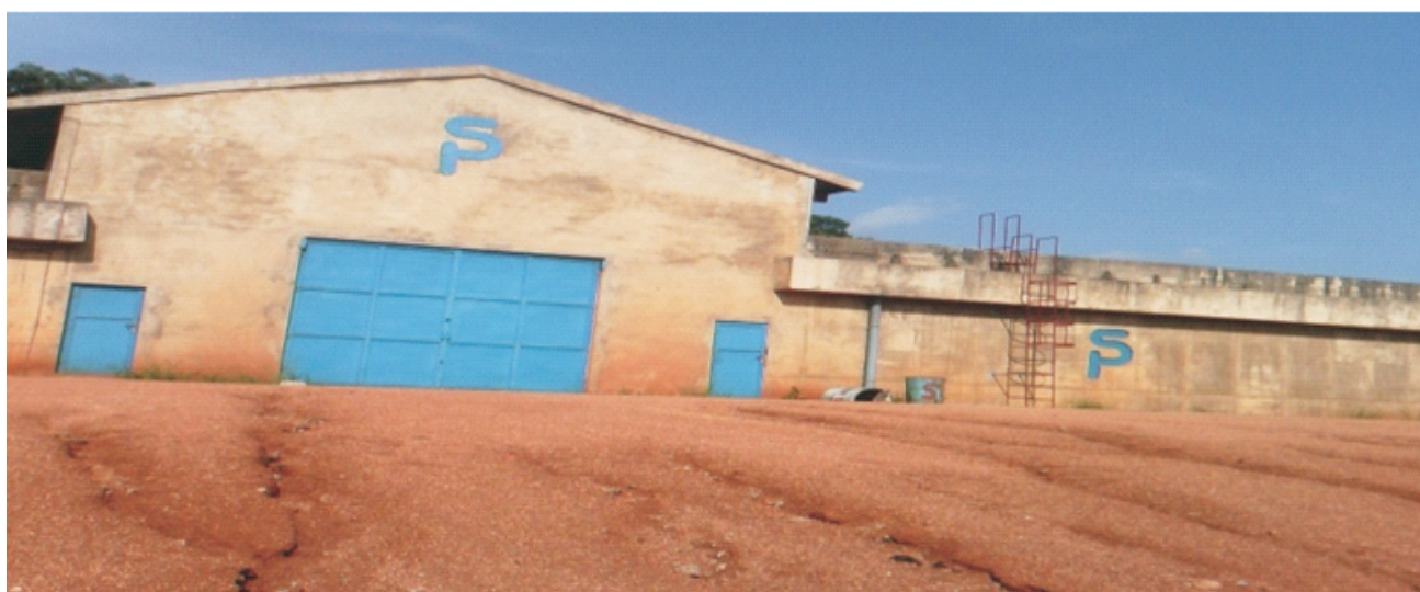
Picture 4: Completed Work of Tank 1 Water Treatment Plant at Dawaki
