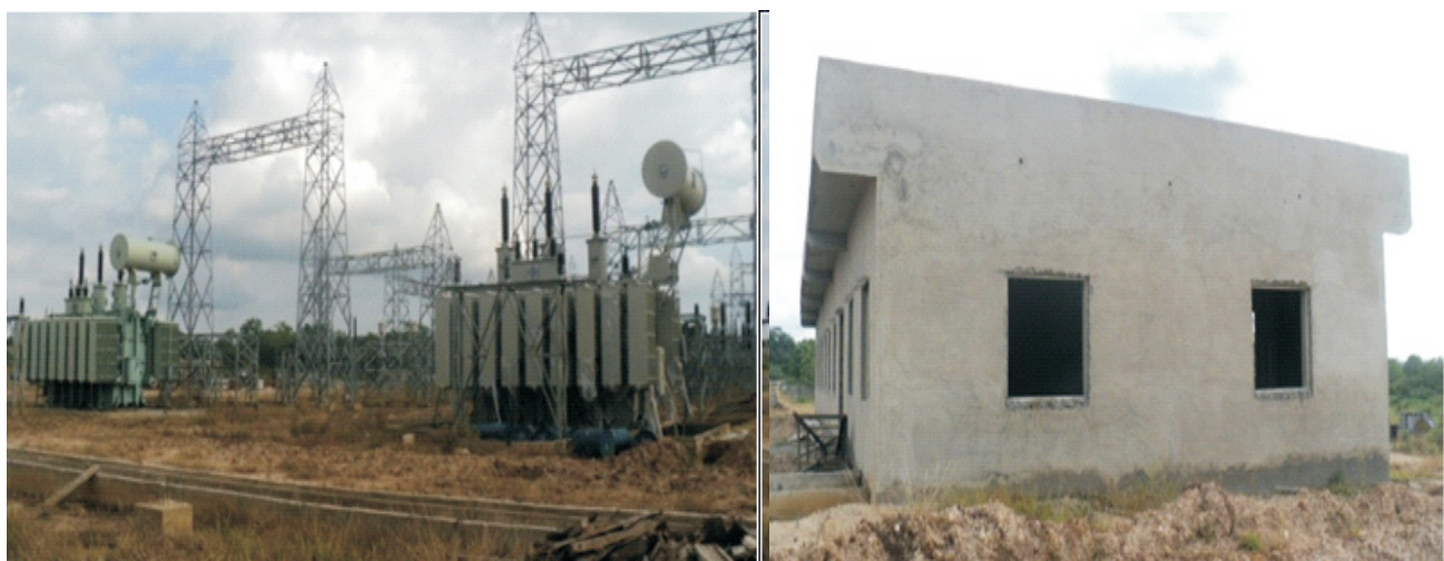
Picture 16: Installation of 2no. 60MVA Transformers & Construction of Control Room in Progress at the Site
