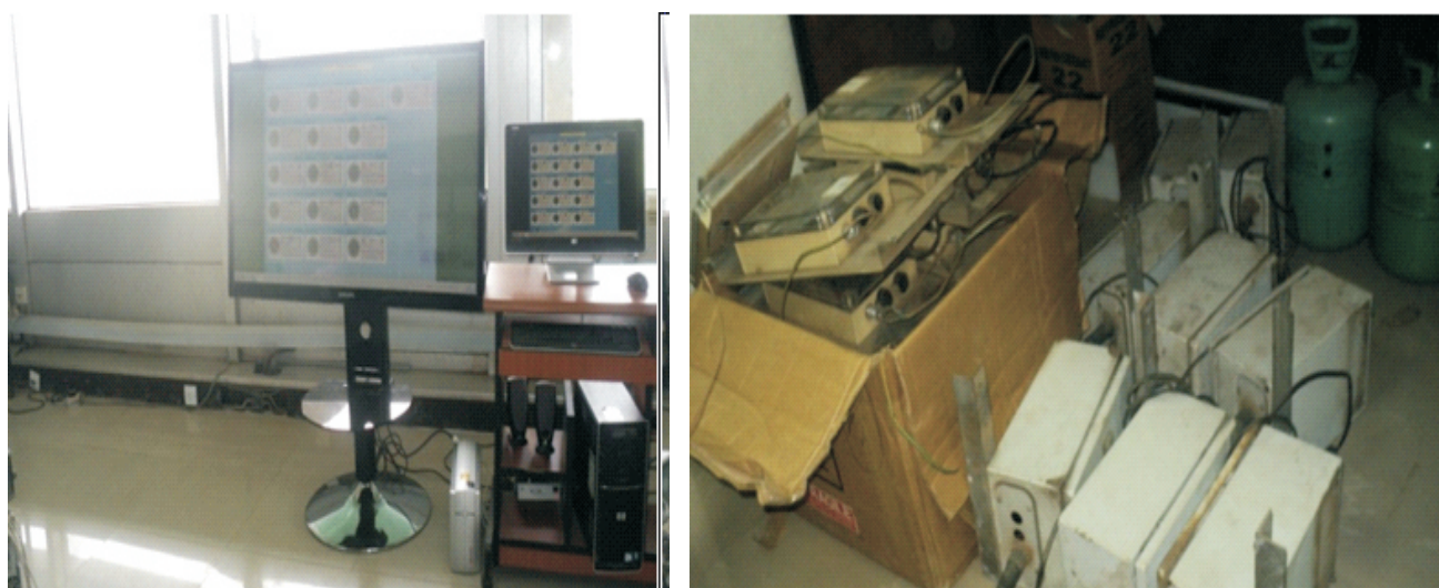
Picture 19: Replaced Spare Parts and Alert Display System at the Lagos International Airport
