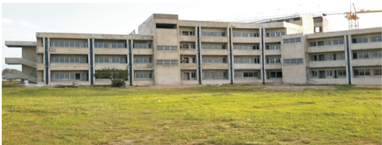
Picture 29: Construction of Administrative Block/Senate Chamber
