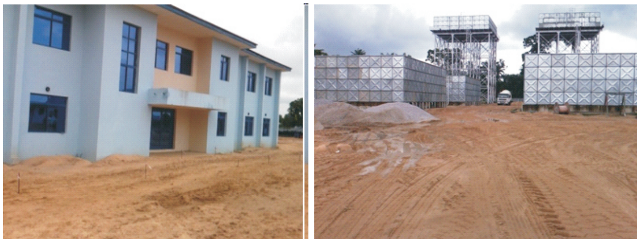
Picture 6: Completed Administrative Building and the Overhead Water Tanks at Ogbia
