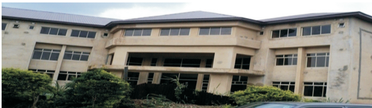
Picture 31: On-going Construction of Consulting Complex at FMC Umuahia
