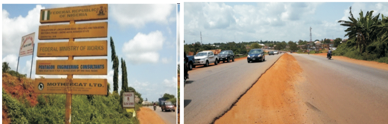
Picture 12: A Completed Portion of the Obajana Junction to Benin Phase 2: Section II (Okene to Auchi)
