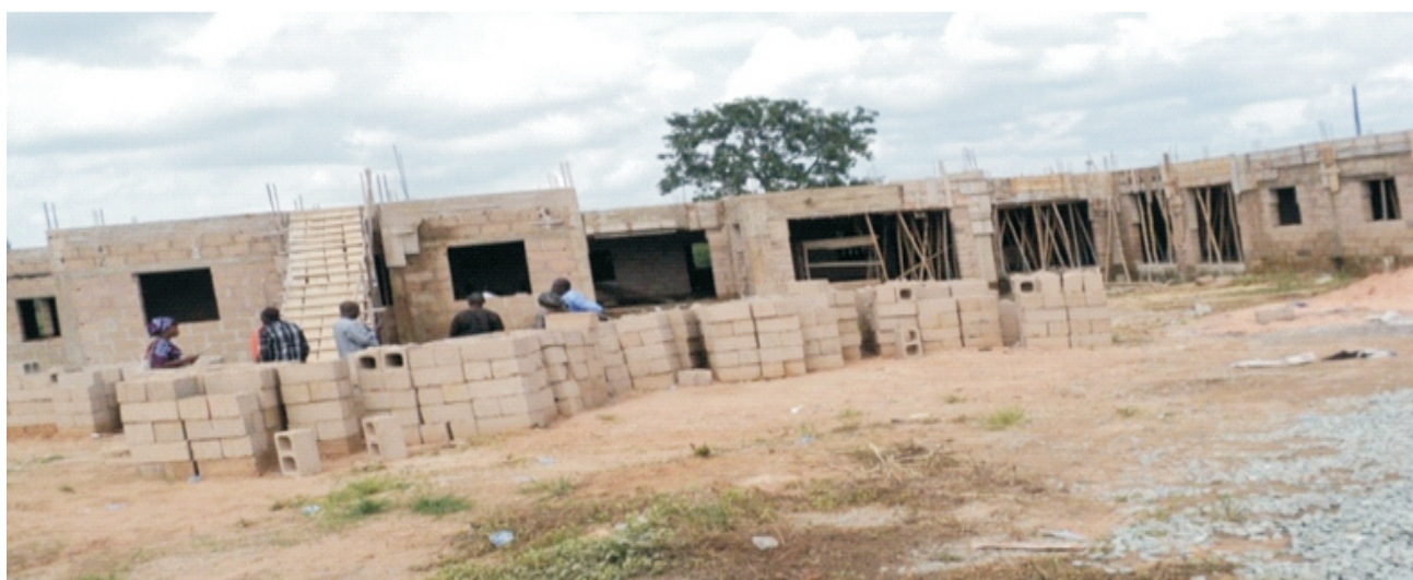
Picture 24: On-going Construction of Lecture Theatre at Federal College of Agriculture, Ishiagu, Ebonyi State
