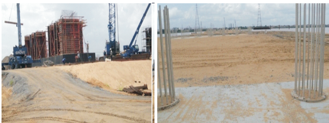
Picture 10: On-going Piling Works, Hydraulic Filling and the Construction of Pile Caps of the 2 nd Niger Bridge
