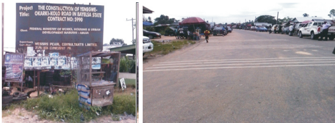
Picture 11: On-going Construction of Yenagoa – Okaki – Kolo Road
