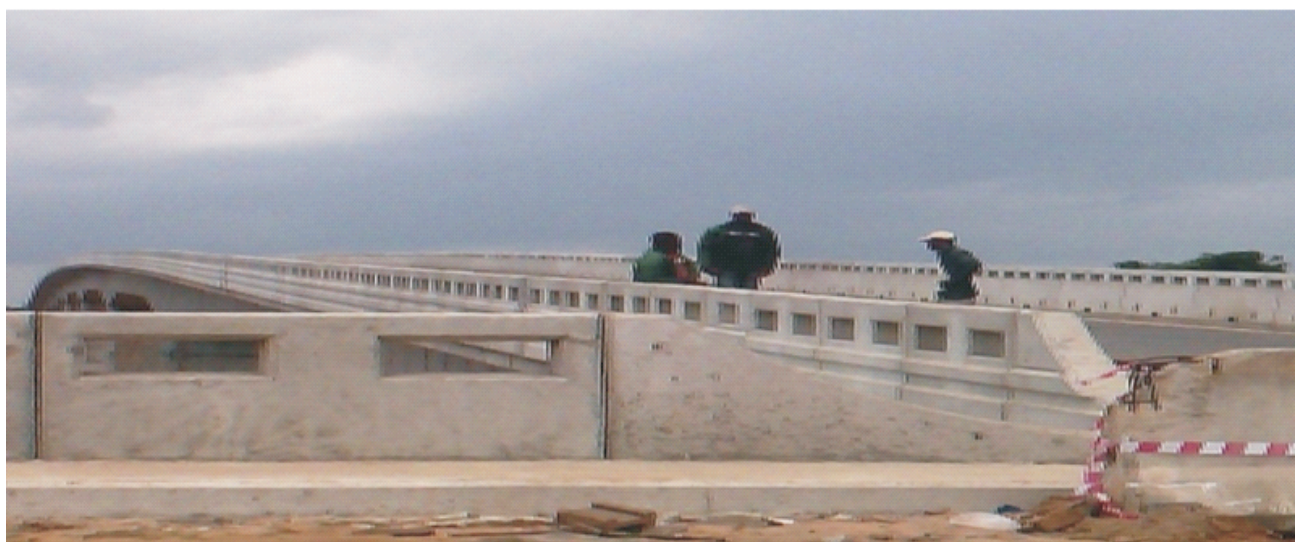
Picture 13: Completed Patani Bridge
