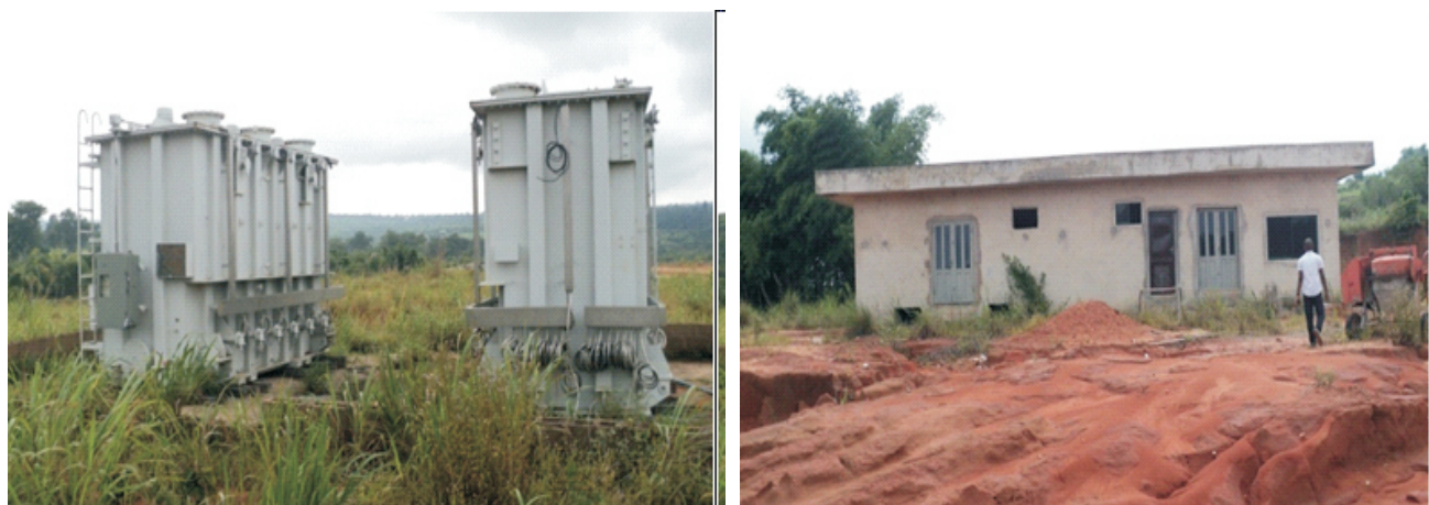
Picture 17: 2x60MVA, 132/33KV Transformers and Constructed Control Building at Project Site at Oba (Ojoto) Anambra State
