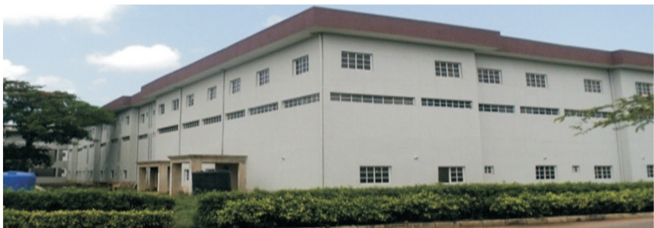
Picture 30: the Operating Theatre Complex almost Completed at the Hospital
