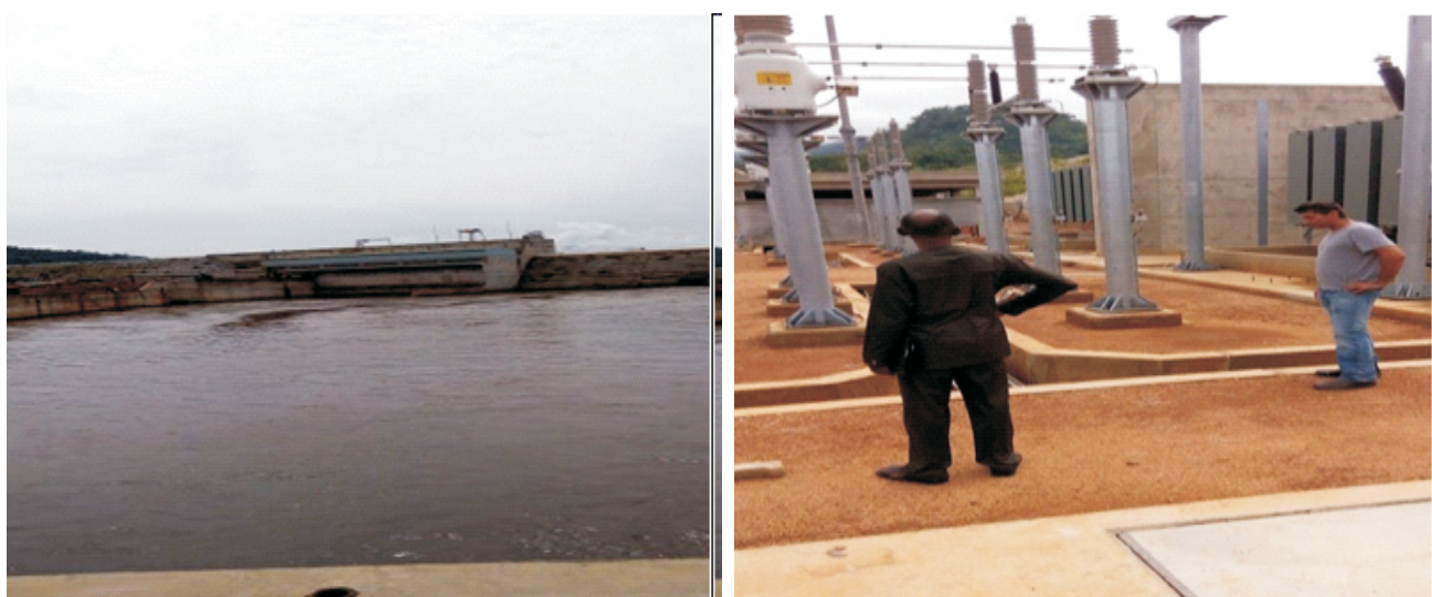
Picture 5: Completed Dam and Switch Yard Substation for Hydropower at Kashimbilla
