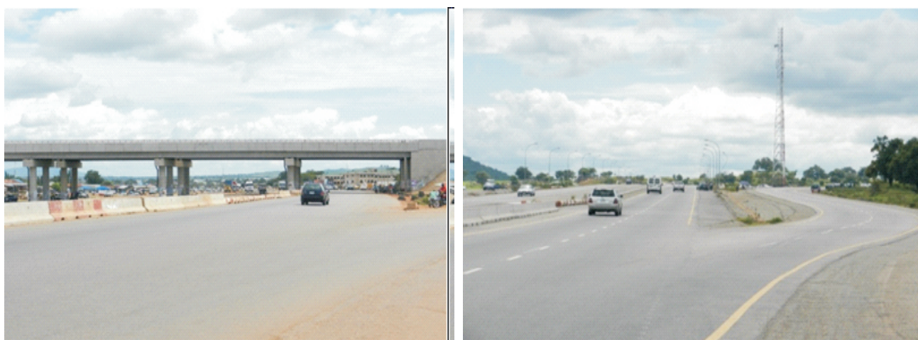
Picture 9: Completed Interchange in Gwagwalada Township & a New Carriageway along the Airport Spur
