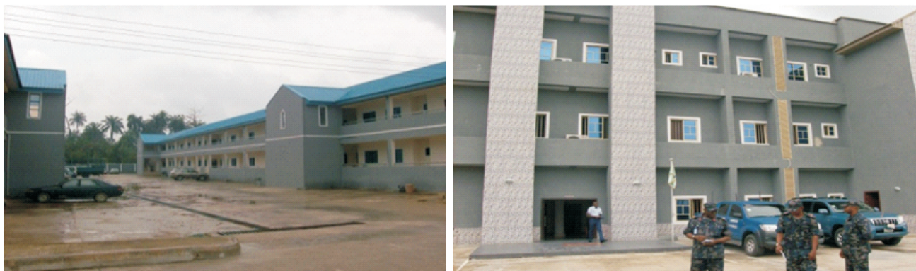
Picture 34: Completed NAF Barrack Residential Accommodation and Mobility Command HQ Office at Yenagoa
