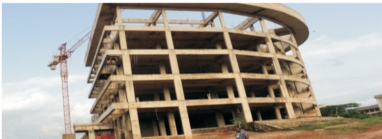
Picture 28: Ongoing Construction of Administrative Building in UNN, Enugu Campus
