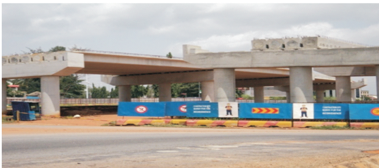
Pictures 1: On-going Construction of Overhead Bridge at Villa Roundabout
