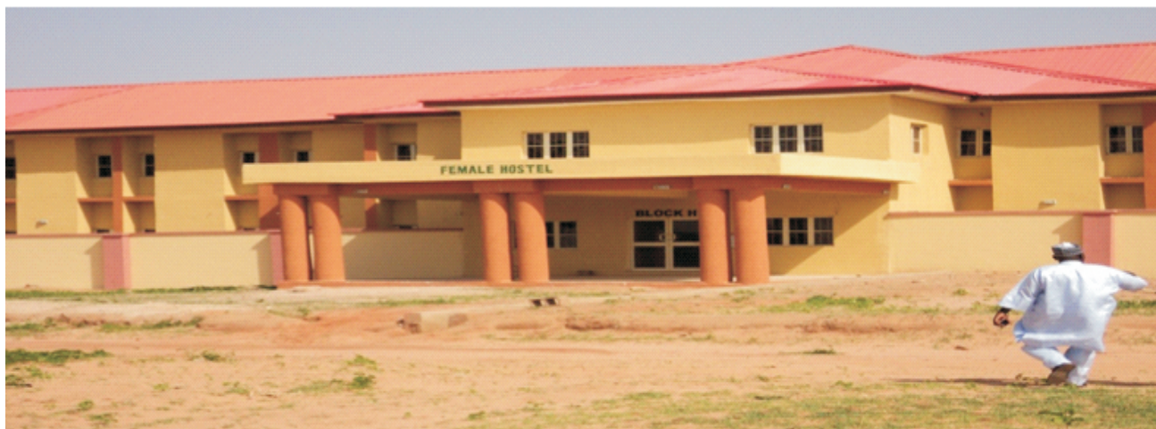
Picture 26: Completed Structure of Female Hostel at FCE, Gombe.
