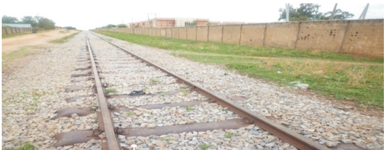
Picture 22: Part of the Completed Stone Pitching at Zaria to Kauran Namoda Rail Track
