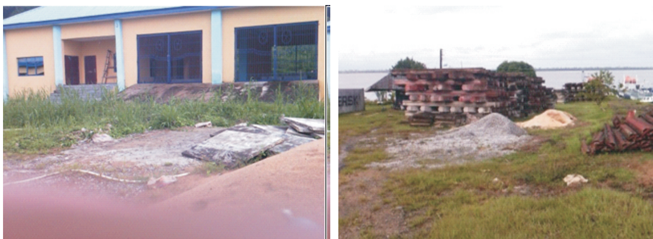
Picture 23: Completed Maintenance Workshop and Piles for the Protection of the Erosion
