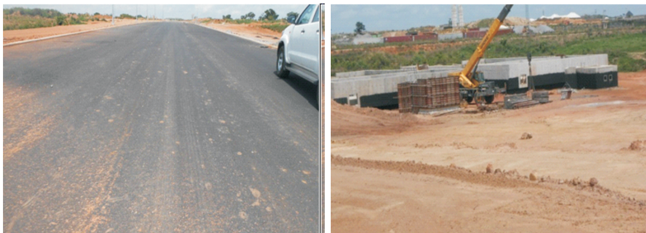
Picture 3: On-going Road Construction and Sewage Treatment Plant (with Completed Structure)
