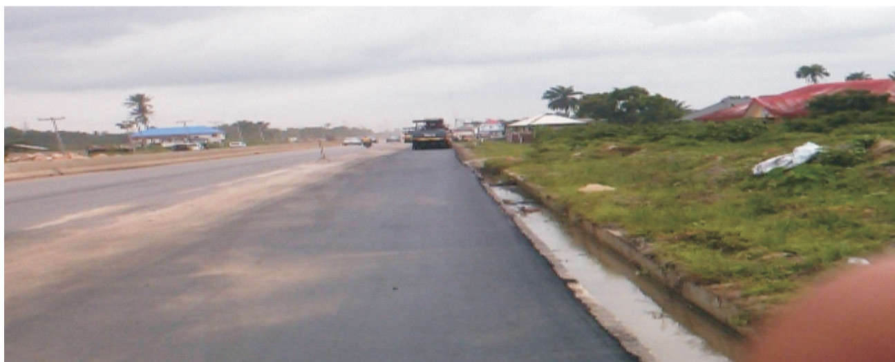
Picture 14: On-going Shoulder Works on Port – Harcourt - Ahoada Road
