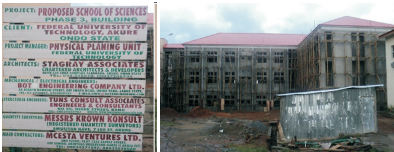
Picture 27: On-going Construction of School of Sciences Building Phase III
