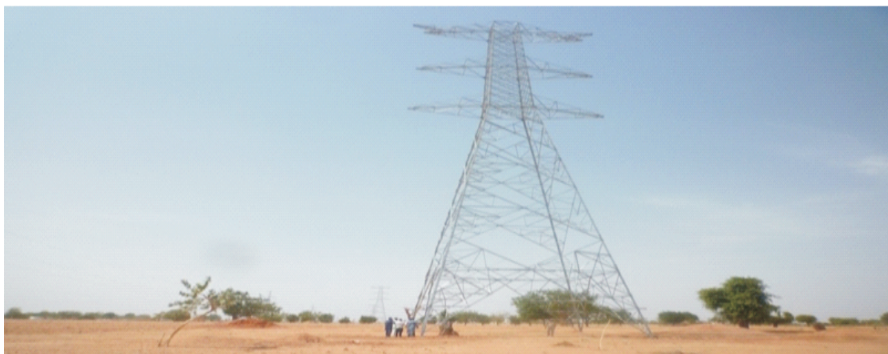
Pictures 18: Erected Tower Type -Stub of D/C Transmission Line Between Kano and Katsina
