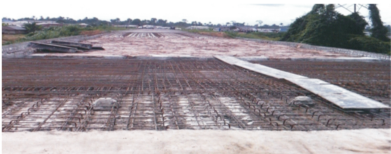
Picture 15: On- going Works at Kiama Bridge
