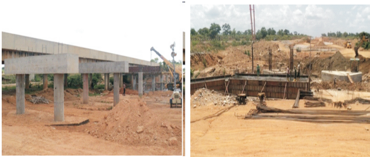
Picture 2: Cross Beams at Layi River Bridge and Pilling Work in Progress at Dnako River Bridge
