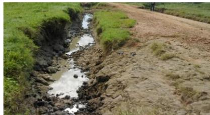
*Eroded road due to deviation culvert not removed*
