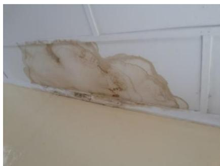
*Stained ceiling board due to leaking roof*
