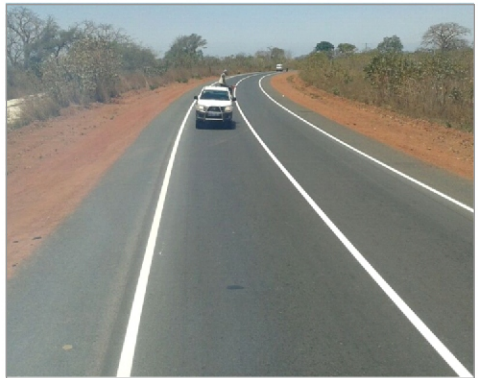
Cross section of Roads - a major leap in opening up the country
