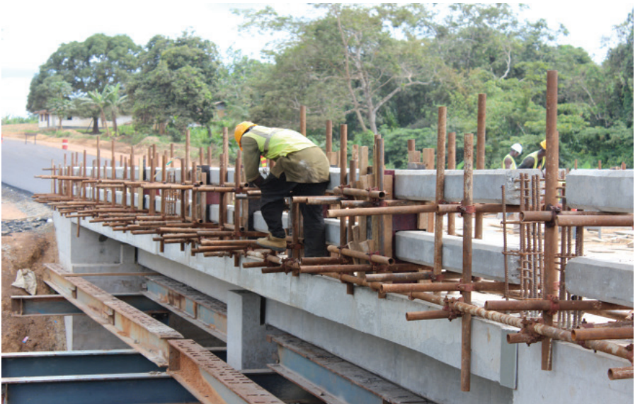
Konola bridge construction (Monrovia - Ganta Highway Project)
