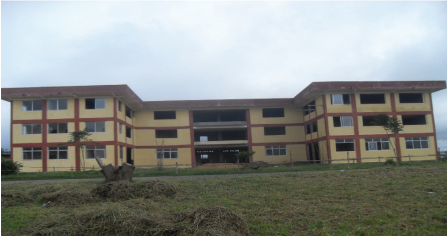
Rehabilitated BWI Technical Building (circa. 2012)
