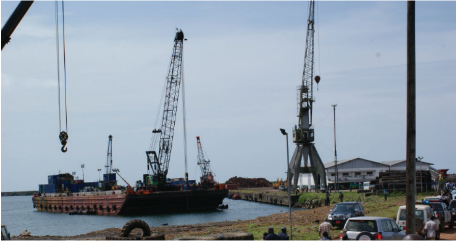
Dredging of the Buchanan Port (circa. 2012)
