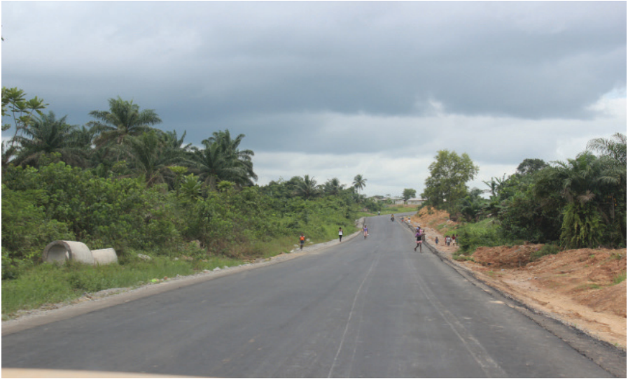
Bong Mines rehabilitated road (2012-2013)
