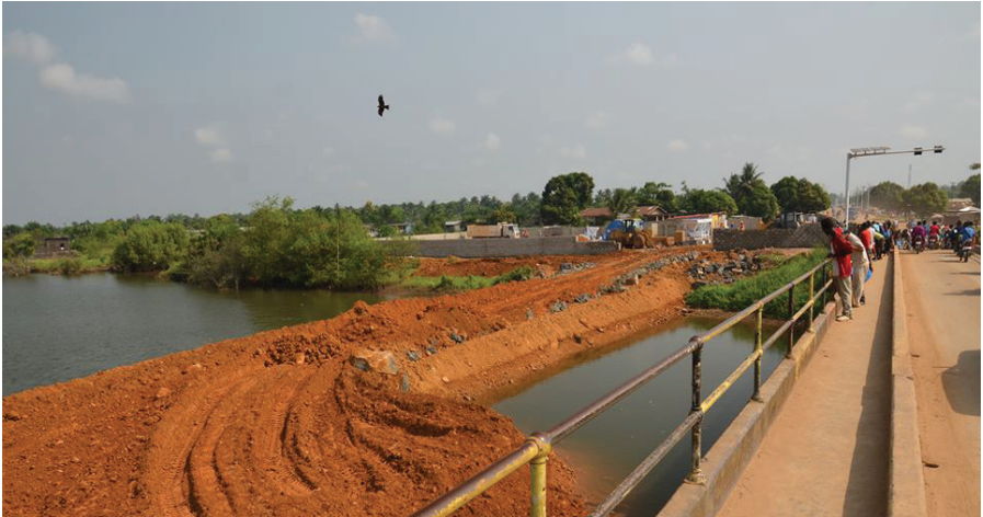
Construction of the Caldwell Road Bridge
