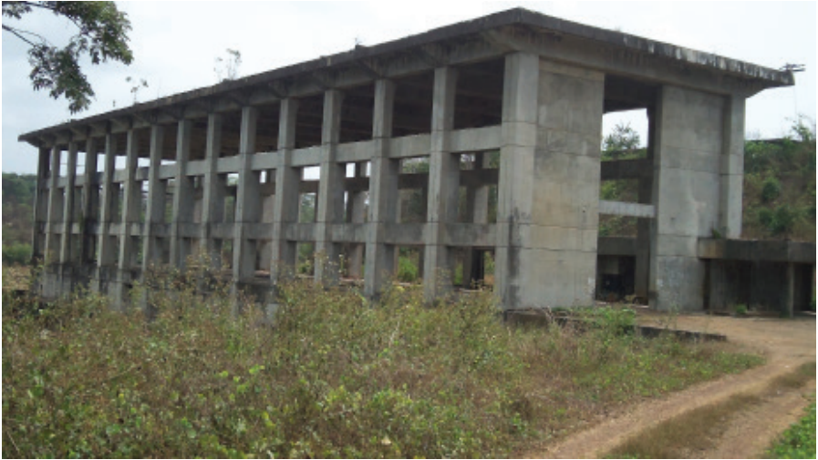
Mt. Coffee Rehabilitation to be completed 2015-2016
