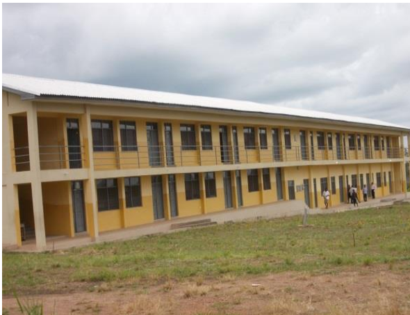
Newly Constructed Classroom Block
