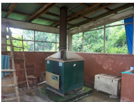
Figure 4 - Defective Incinerator at Connaught Hospital
