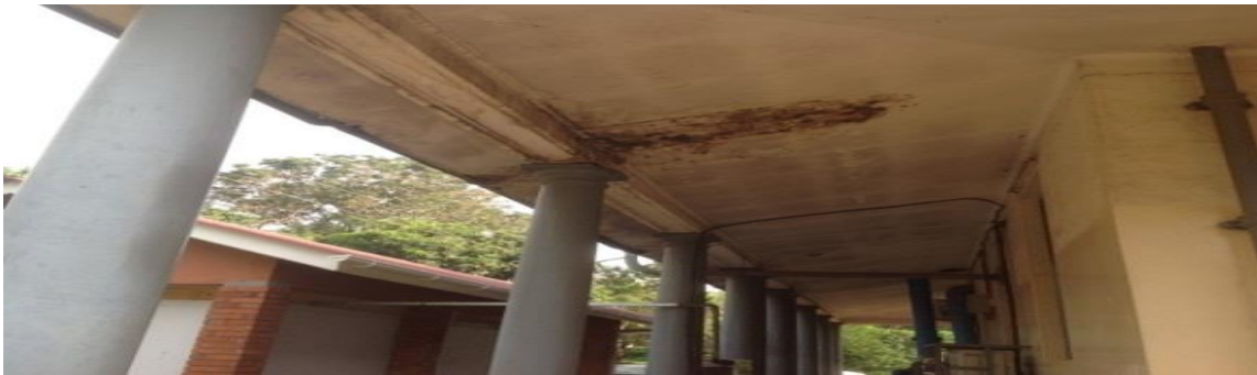
Leaking ceiling that needs urgent repairs/renovations
