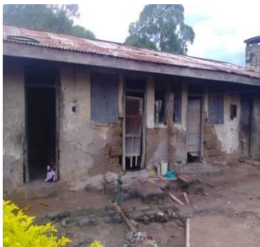
Dilapidated house in Arua
