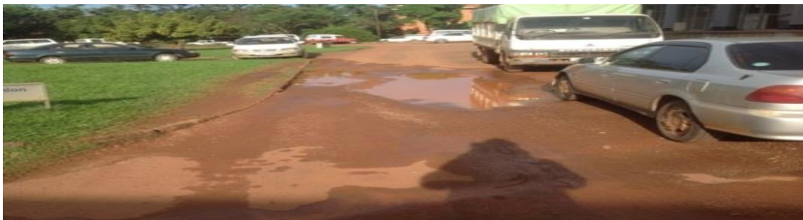
Front parking with big potholes filled with water.
