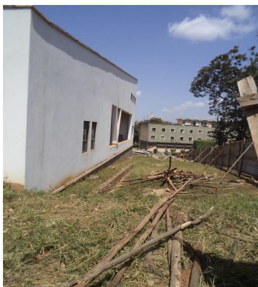
The side view of the auditorium.
