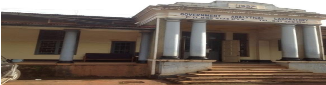
Main entrance of the directorate headquarters: Falling facial boards; Stairs in a sorry state; Building looks abandoned
