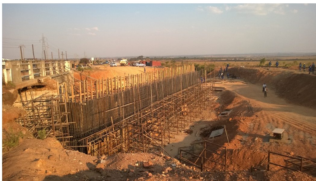
Mabvuku road over rail bridge
