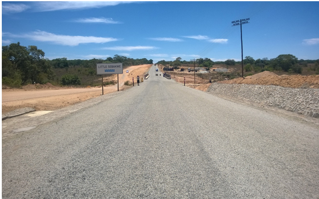
Completed Little Sebakwe Bridge and Approaches, on Chivhu-Nyazura Highway
