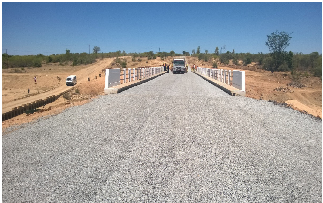
Musavezi Bridge , Department of Roads conducting final surfacing, on Shurugwi-Mhandamabwe Highway
