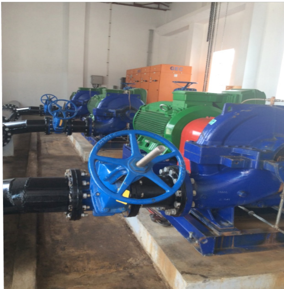
The three KSB pumps, with capacity to pump 720 cubic metres per hour were commissioned at Mtshabezi Pipeline Project by the Vice President, Hon E. D. Mnangagwa on 17 October 2015.
