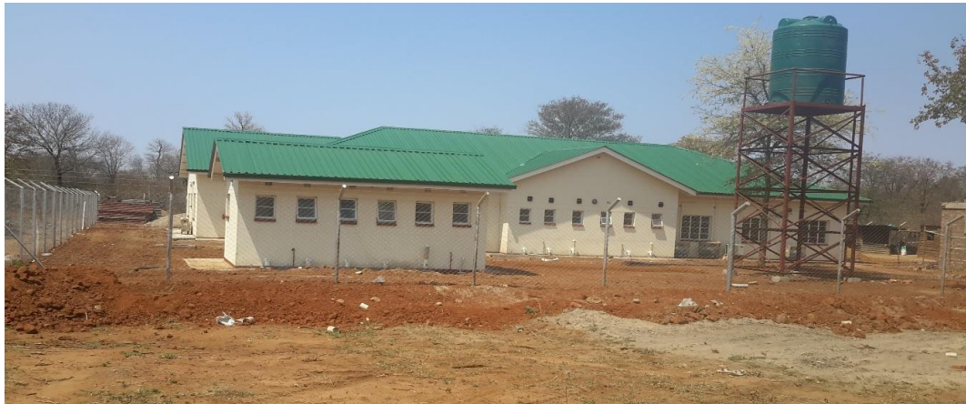
A typical Court House with Legal Aid Offices, Victim Friendly Room, Child Testimony Room & Access ramps for disabled persons, built by the Royal Danish Government
