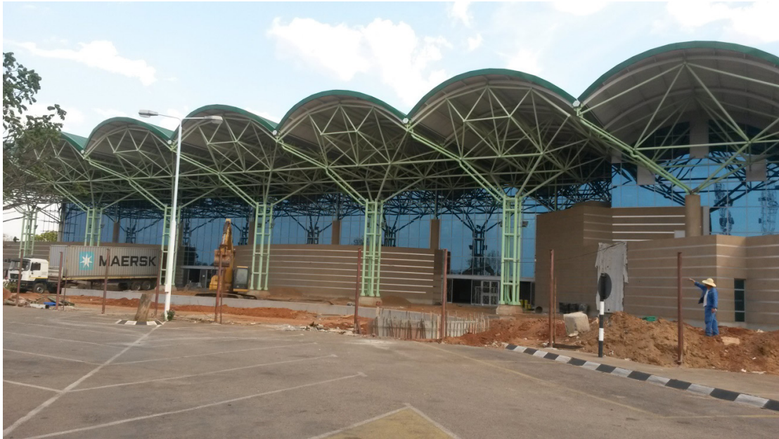
The new Terminal Building at Victoria Falls Airport, expected to be commissioned before year end.
