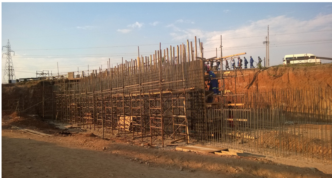
Mabvuku road over rail bridge
